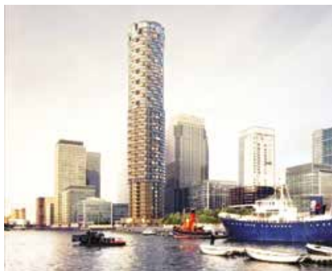
Wood Wharf, Canary Wharf, London, United Kingdom
