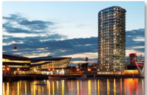
Pump Tower Royal Victoria Dock, London
