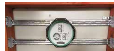
A Hansgrohe iBox shower valve installed using BK4 brackets.
